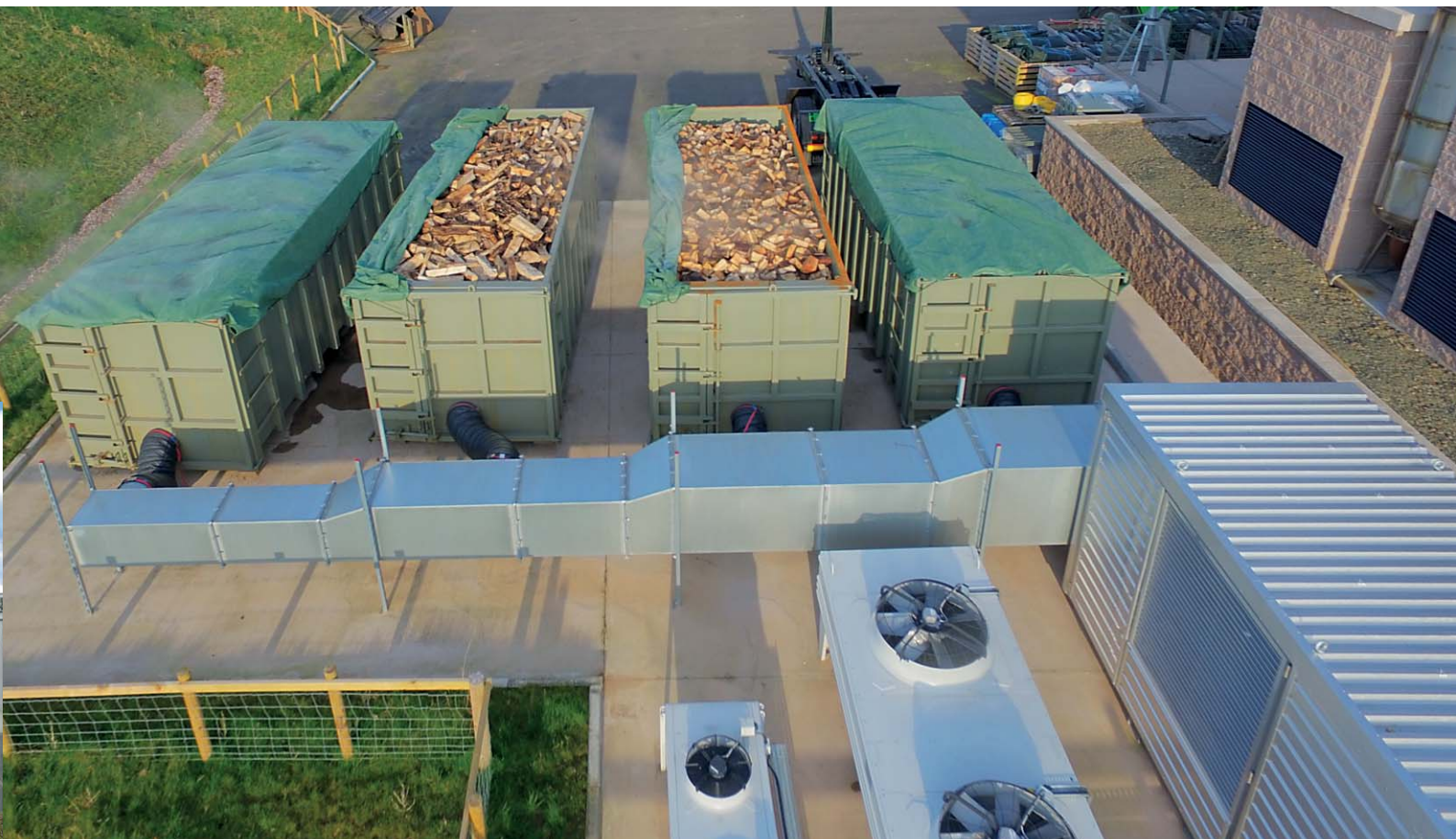
Biogas plant in England with a L-ENZ 370, air duct and four drying containers.
