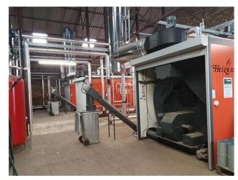
The solution we provided was to supply 3 Heizomat RHK-AK 1000 (990kwh) biomass boilers and 20,000L hot water storage tank for each boiler. One of the boilers was used to supply heat to the grain dryer the improved output increase production of dried grain immediately. The other two boilers were installed with additional drying floors that could be used for wood, animal bedding or grains. (The drying floor option has the future proofing of a diverse range of product options)
